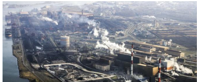
Picture 10: ArcerlorMittal Dunkerque Source: Laurent Grandguillot
