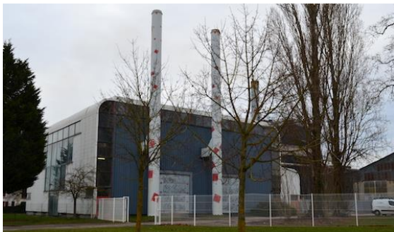
Picture 15: Wood-fired heating plant Vitry le François. Source: Frédéric Douard
