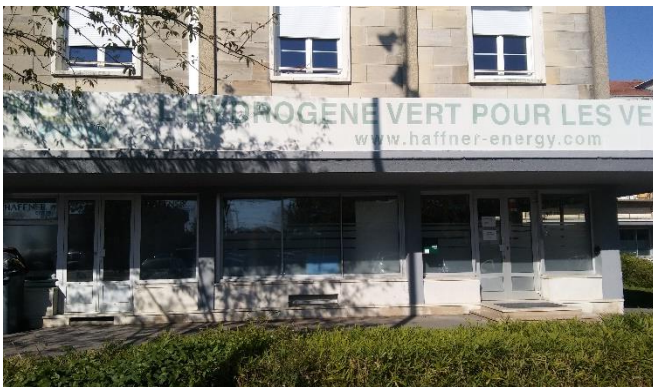
Picture 36: Haffner Energy Headquarters in Vitry le François. Source: Author, Vitry le François, 2021
