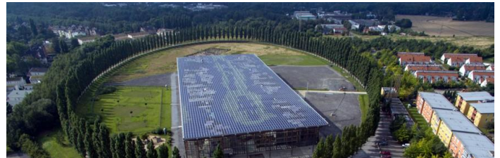
Picture 2: Energy Park Mont Sant - Cenis, Herne. Source: StadtHerne
