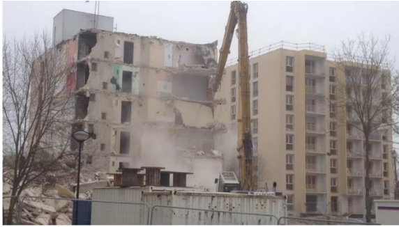
Picture 17: Demolitions in Le Hamois neighbourhood. Source: Elodie Vergelati.
