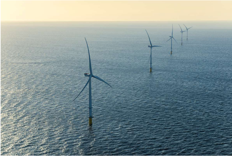
Figure 2.5. V164-9.5 MW turbines from MHI Vestas Offshore Wind [136]
